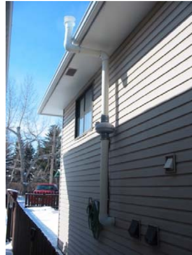
Figure 6: Typical fan and pipework configuration for depressurisation system
