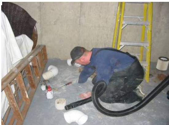
Figure 8: Construction of internal sump
