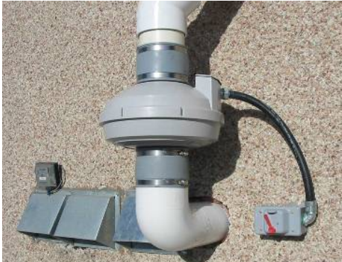
Figure 5: Typical fan for sub-slab or crawl space depressurisation
