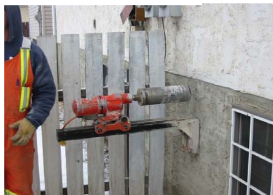
Figure 9: Construction of external wall penetration
