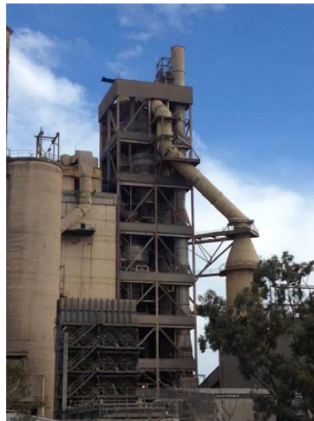
Pre-Calcliner Plant Stack (Stack 4B)
