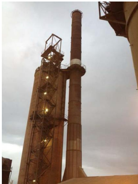
Dry Process Kiln Stack (Stack 4A)
