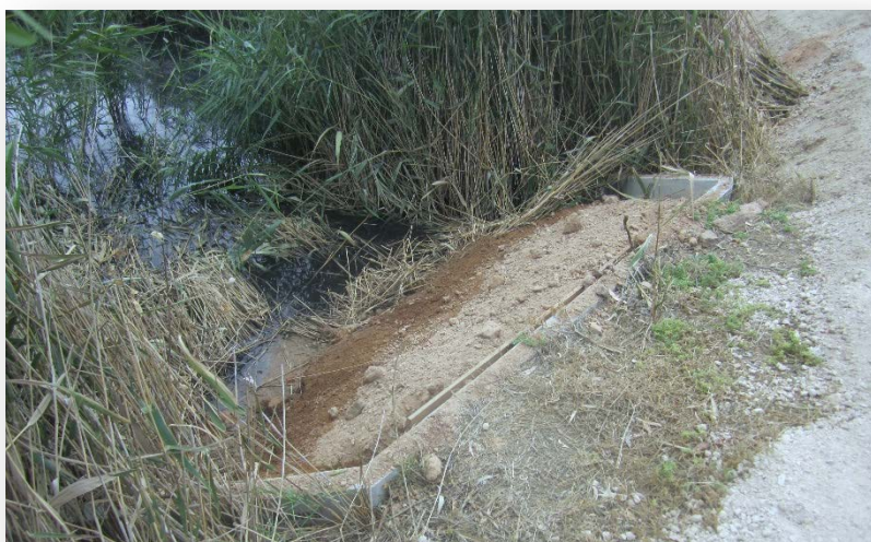
Culvert sealed by the EPA on 4 January 2018 to prevent fire water discharge.
