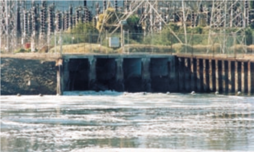
Cooling water is discharged from the Torrens Island power station into the Angas Inlet.
