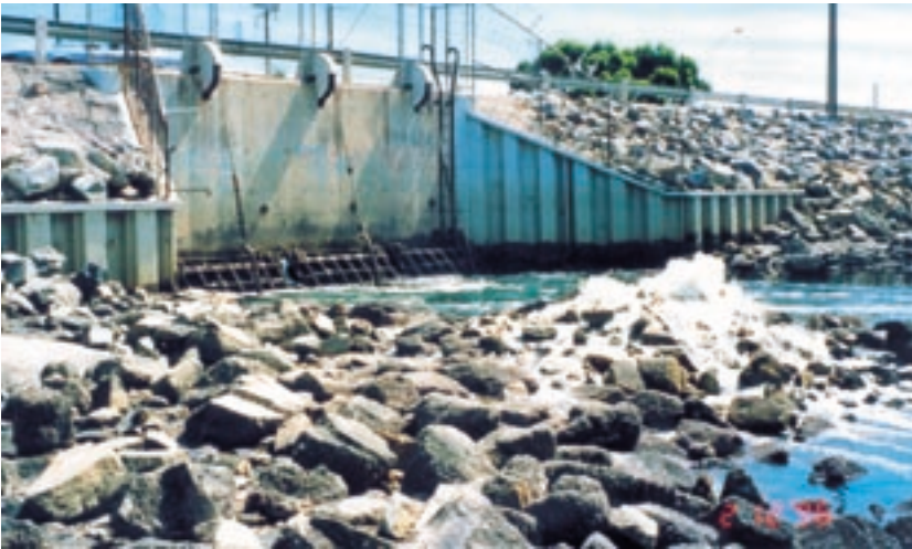
The Port Adelaide wastewater treatment plant discharges treated effluent into the southern end of the Port River, by the West Lakes tidal outlet gate.
