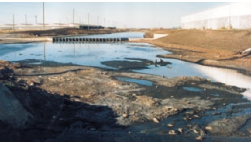
A trash rack and a newly designed wetland system are designed to improve the quality of stormwater before it is discharged into the Port River.
