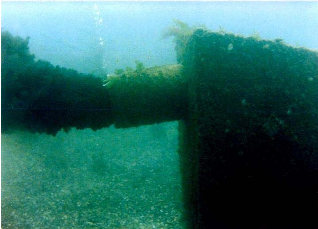
Figure 2. The Port Adelaide WWTP digested sewage sludge outfall, discharging 4.5 km off Point Malcolm (Photo by: V. Neverauskas).
