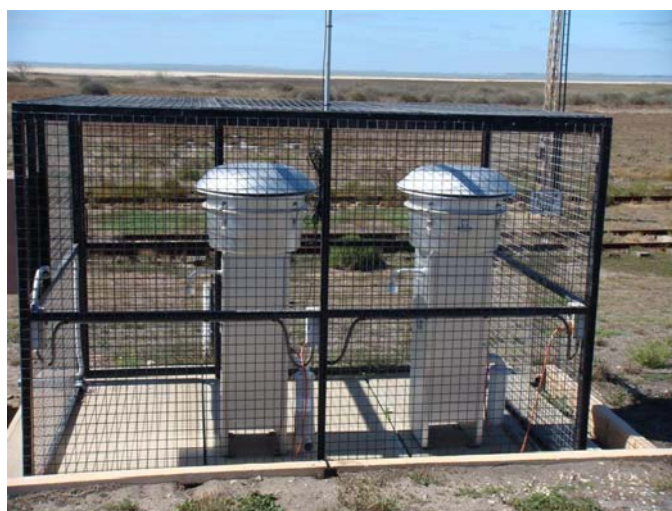
Figure 5 Two HiVol units (one wind switched and one 24-hour) installed at Milang
