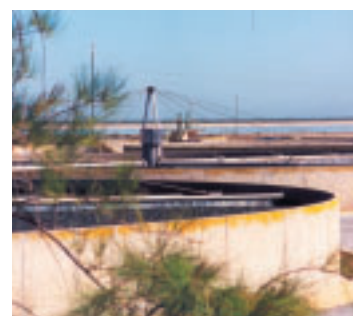
Bolivar sewerage treatment tanks
