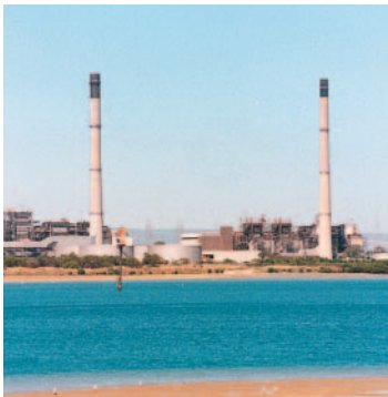
Torrens Island powerstation
