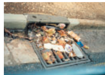
Litter clogging a street drain on West Terrace, Adelaide Photo Tony Jones, courtesy KESAB Environmental Solutions
