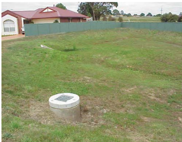
Figure 25 Retention basin with gravel trench floor and gravel surround at bore
