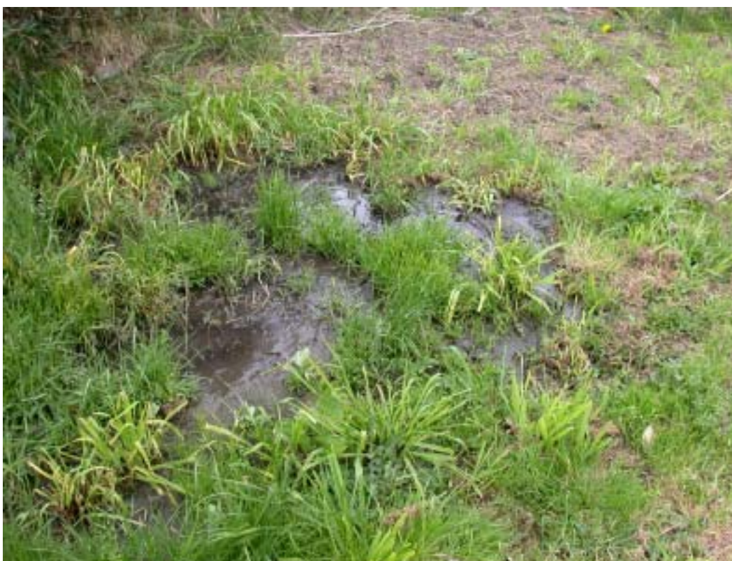
Plate 7 Effluent leaving a septic tank in the Lenswood Creek sub-catchment
