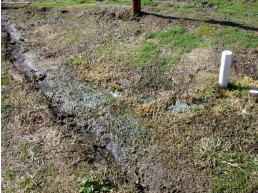
Plate 4 Overland wastewater flow from septic tank on Coleman Road
