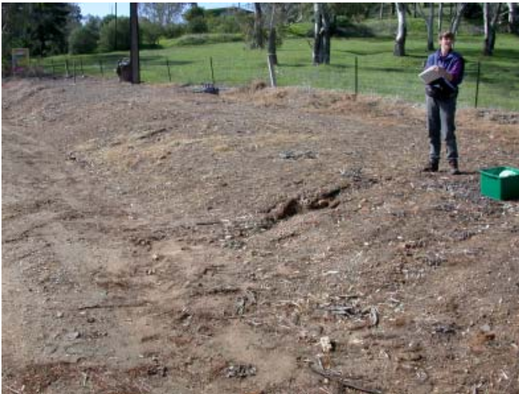
Plate 10 Roadside drain at Williamstown (Victoria Creek sub-catchment)
