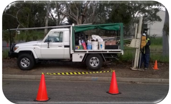
A soil vapour bore being drilled on a road verge
