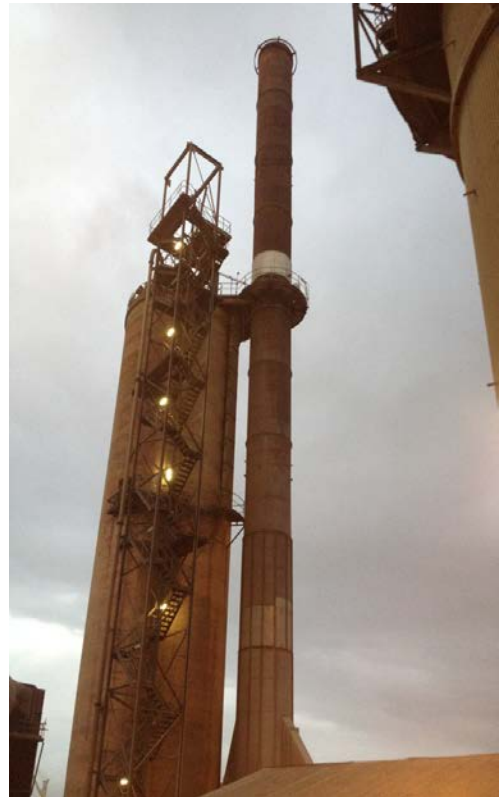
Figure 1: Kiln 4 Main Stack (RP 4A)
