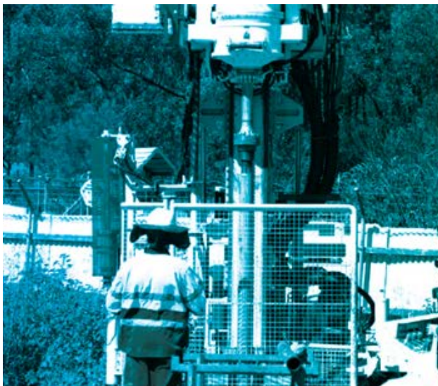
Drilling groundwater sampling well
