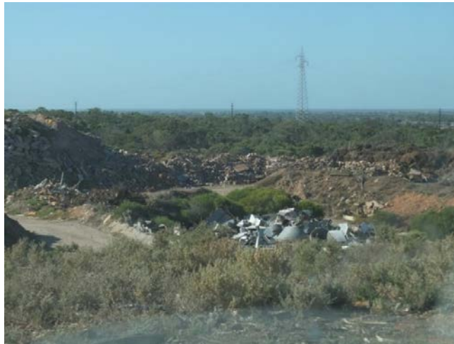
Large stockpiles of mixed waste derived from construction and demolition waste (with a scrap metal stockpile in the foreground)
