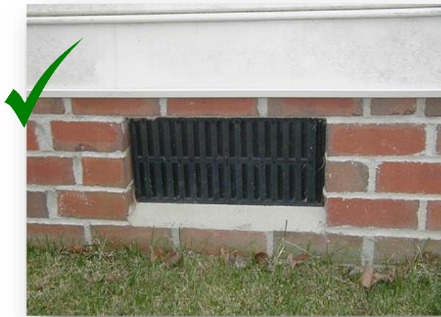
Clear vents allows maximum airflow
