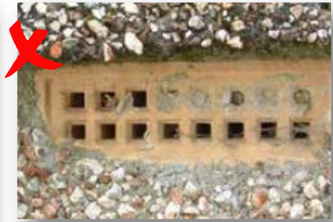
Replace older vents with newer vents
