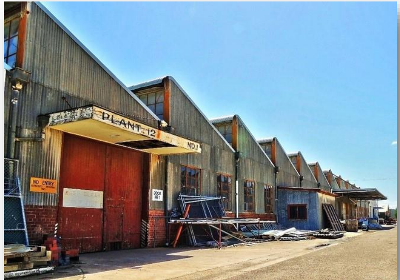
Finsbury Munitions Factory Building later used as an Email household goods parts centre, photo courtesy of Dave Walsh
